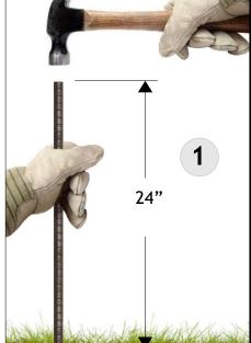
Use hammer to drive rebar into ground. Leave approximately 24" above ground.
