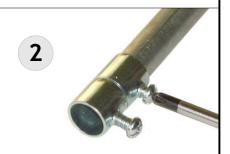
Attach 1/2" EMT coupler to end of conduit. Tighten upper screw against conduit. Install longer screw in bottom but do not tighten.
